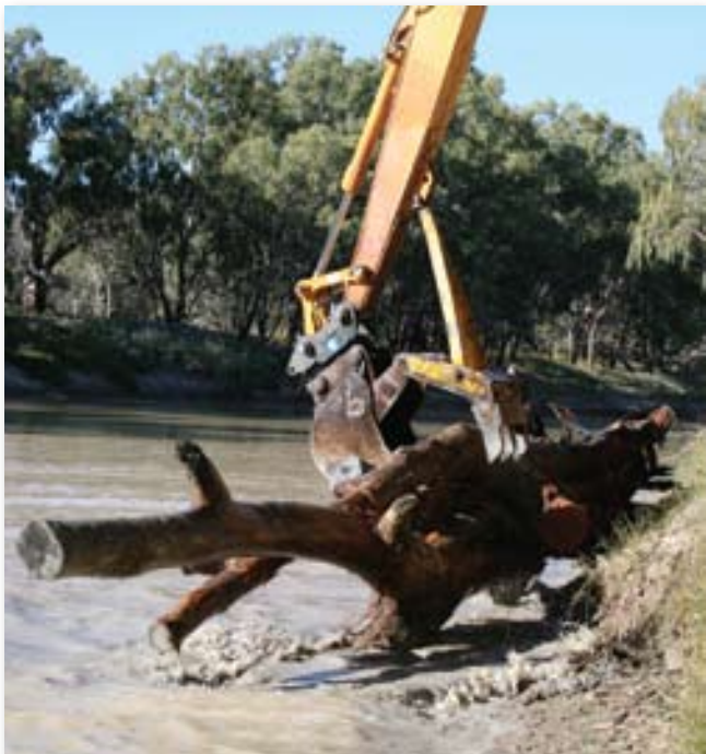
The Western CMA and Industry and Investment NSW have undertaken large-scale re-snagging between Brewarrina and Bourke and near Wilcannia to increase numbers of native fish.
